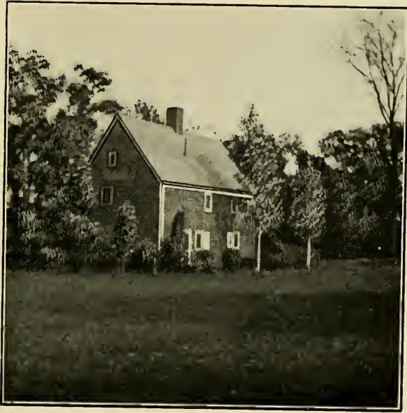
Cottage Street, near Columbia Road
